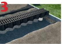
Knockout channel base for outlet and start to lay channels from outlet position.
