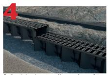
Continue to lay channels working away from outlet, channels slide-fit together.
