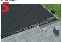
Pour 4" concrete around channel sides allowing for pavement detail (see section drawing above).
