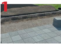
Excavate area to accommodate trench drain and 4" concrete surround.
