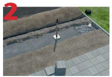
Rough in 3" or 4" SDR pipe or 4" schedule 40 outlet pipe, compact excavation base and lay 4" deep concrete bed.
